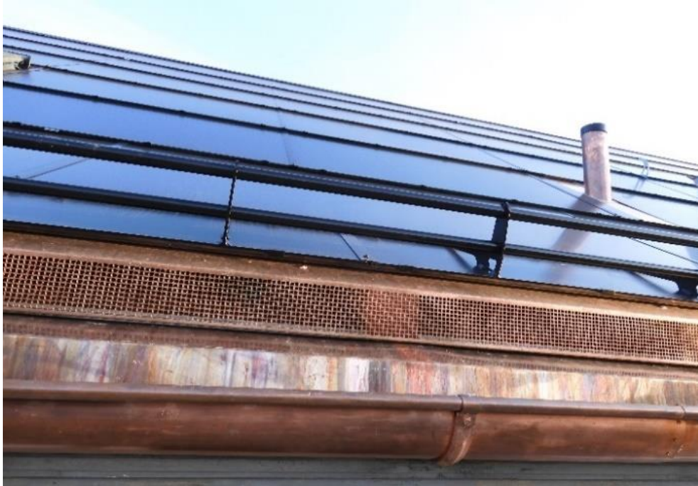
Air intake grille above the rain gutter in the solar roof
