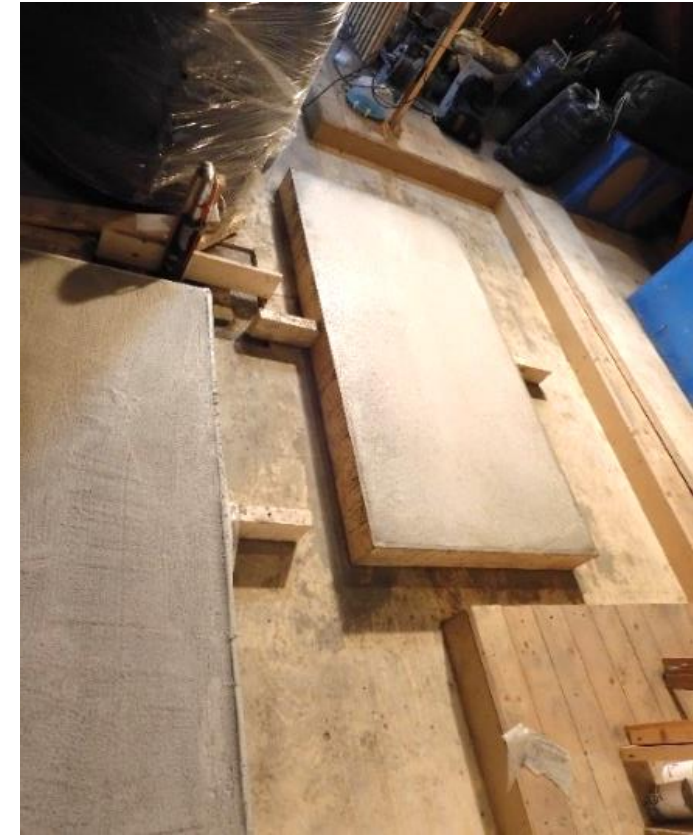
Concrete foundation for HP
