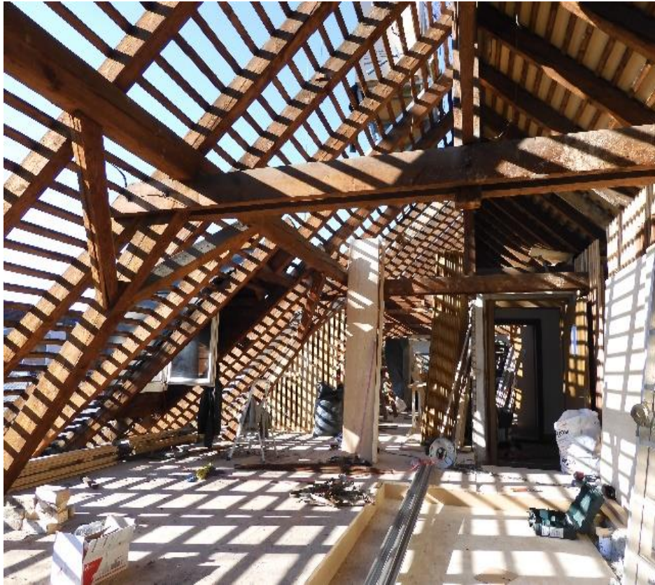
Attic after demolition of the chimneys
