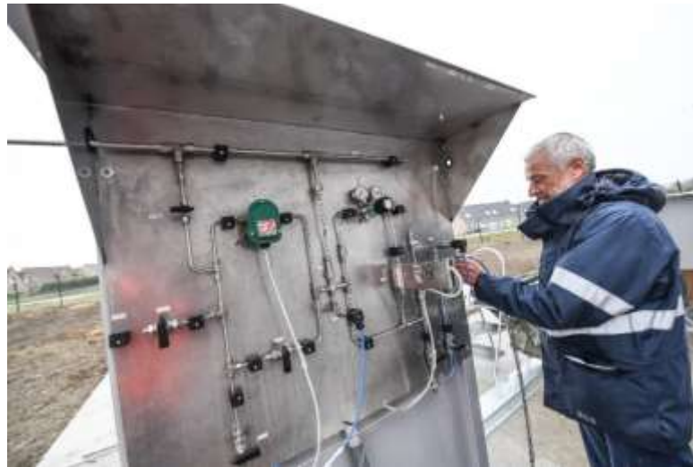
McPhy Energy Stockage H2 solide (hydrures métalliques) 5 kg H2
