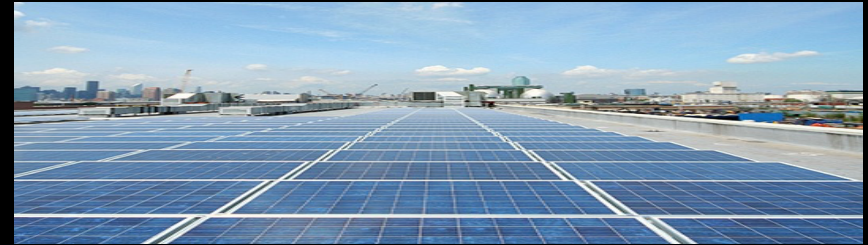
PV PANELS ON THE ROOF
