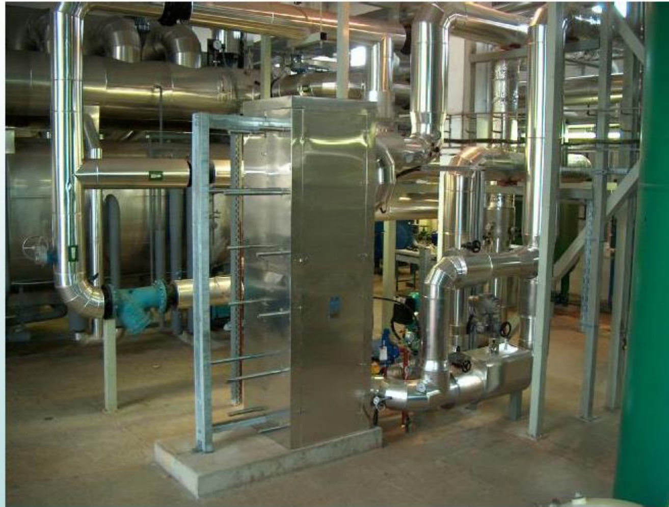
Heat exchanger between district heat supply network and intermediate loop
