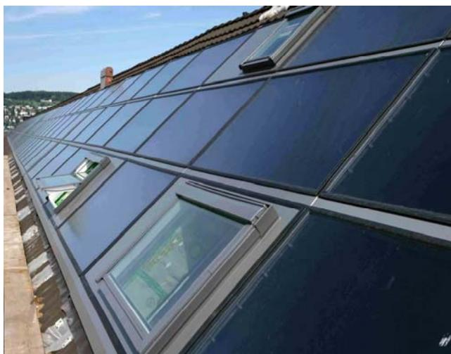
Favorable conditions for applications of glazed PVT collectors are systems with low solar fractions, that means low operating temperatures as in large multi-family houses.
