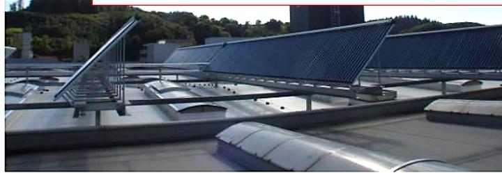
The European-wide operating indoor climate specialist Zehnder launched a 400 m<sup>2</sup> large solar thermal process heating plant in mid-July. The facility is installed on the roof of a new logistics hall in Gränichen, Switzerland and supplies 110 °C hot water for the heat storage of the adjacent paint shop. The solar facility was installed by
